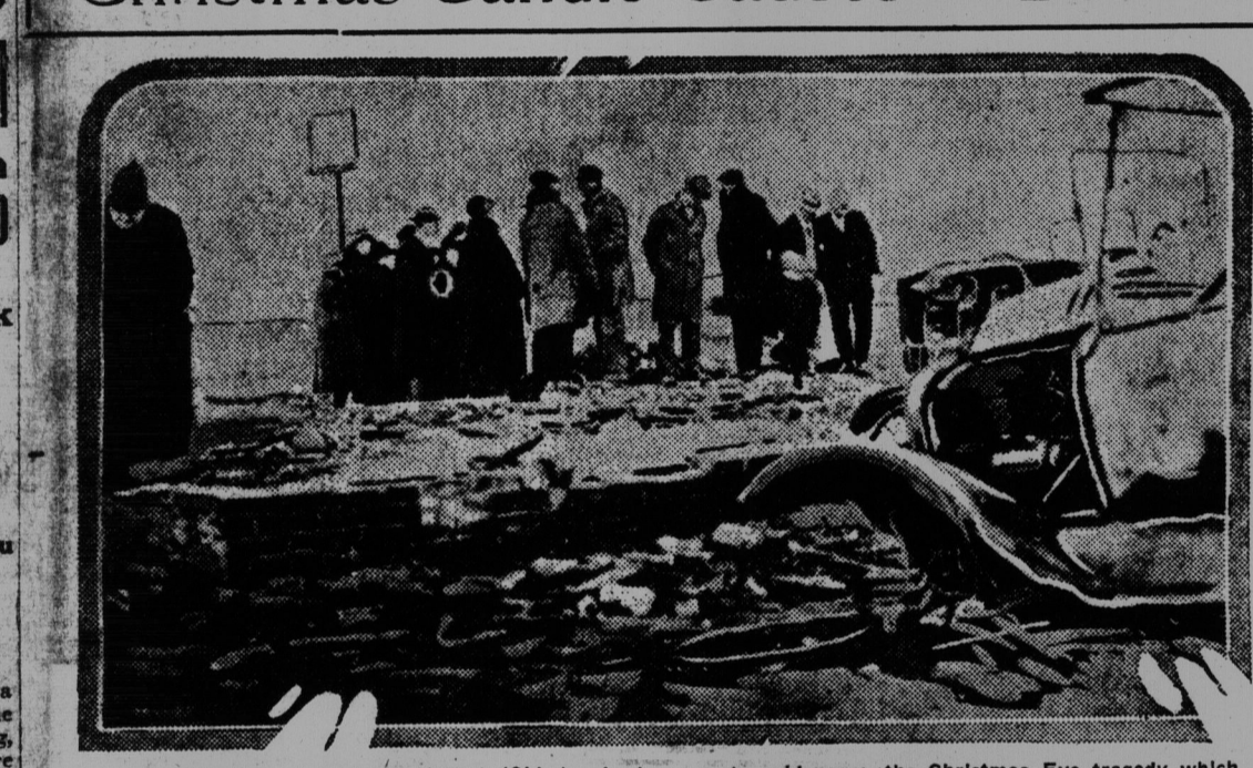
Smoldering ruins of the Hobart (Okla.) school are mute evidence of the Christmas Eve tragedy which caused the death of more than 30 persons when the building burned to the ground.
