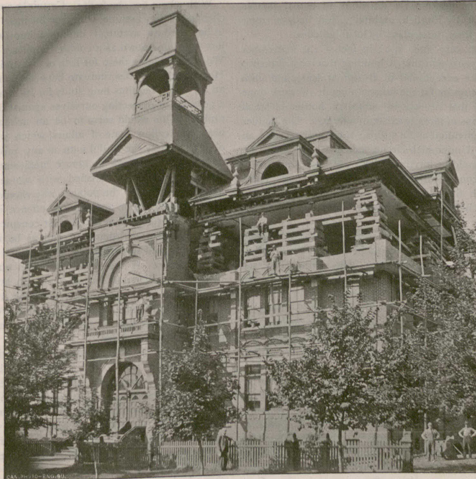
PROCESS OF RAISING THE ROOF, QUEEN VICTORIA SCHOOL, PARKDALE.
