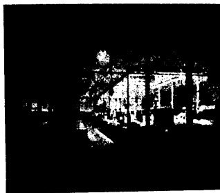
Before Luxfer Prisms Installed.
