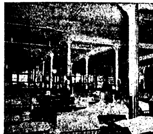
After Luxfer Prisms Installed.
