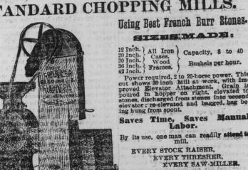
SIZES MADE: Inch. All Iron Capacity, 8 to 40 Inch. Wood Inch. Frames. Bushels per hour. Power required, 2 to 20-horse power. This cut shows 30 inch Mill at work, with Improved Elevator Attachment. Grain is poured in hopper on right, elevated to stones, discharged from stones into second elevator; re-elevated and bagged, hag be-Saves Time, Saves Manual Labor.
