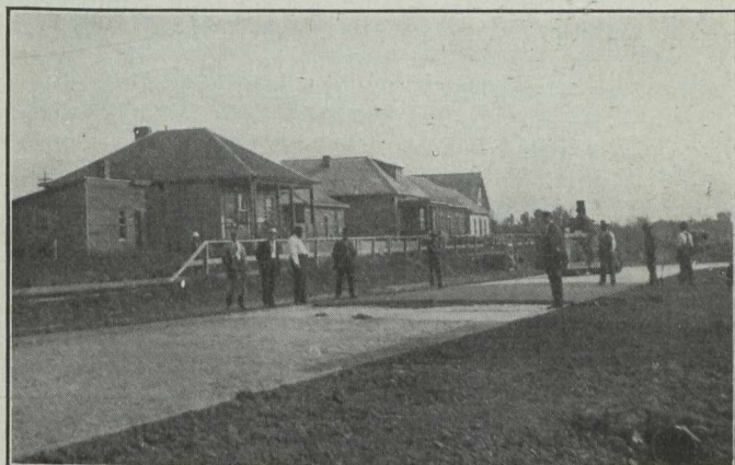
Experimental pavement at Edmonton, laid under direction of S. V. Ells, of the Mines Branch, to demonstrate use of Alberta's bituminous sand deposits.
