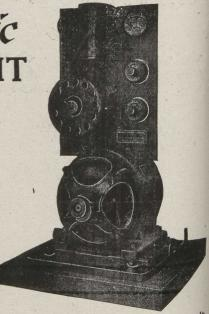
Northern Electric S-8 Belt-driven, 32 volt Electric Plant
