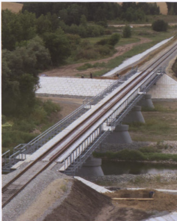
The railway bridge over the Miass River was completed in September 2007.
