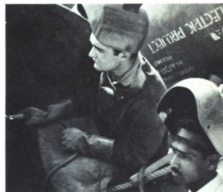
Canadian and Indian welders at the Kundah Dam in India.
