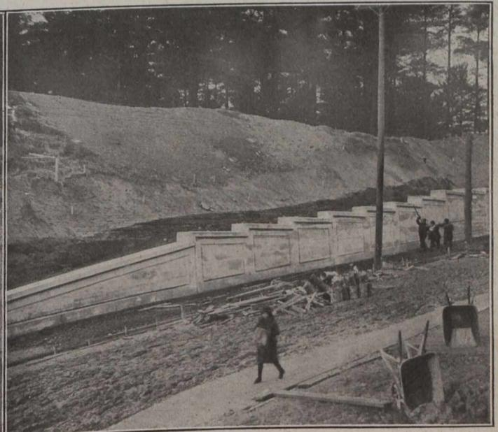
West Wall—Concrete Gravity Section.
