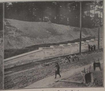
West Wall-Concrete Gravity Section.
