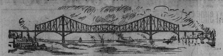
Is Now Under Construction—Will Cross the St. Lawrence River at Quebec—Main Span is 1800 Feet Long and Contains 10,000 Tons of Steel—Cost of the Bridge is \$4,500,000.
