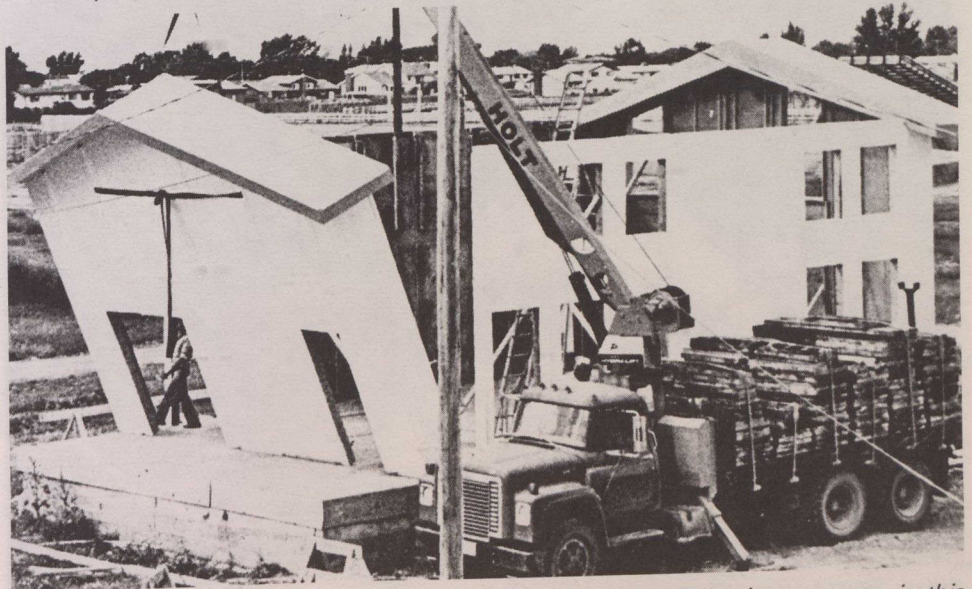
Among the projects supported by the housing technology incentives program is this moulded fibreglass house believed to be low cost and energy efficient.
