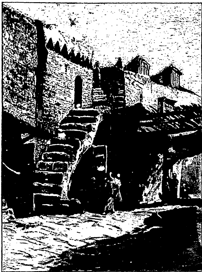
OUTSIDE STAIRS TO FLAT ROOF.
