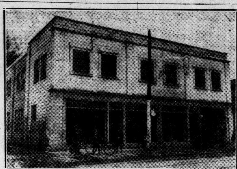
$7,000 DAMAGE IN SUNDAY FIRE. Tennant & Wilkinson's Garage, York street, was damaged by fire caused by an exploding oil heater Sunday morning. Fifteen automobiles were also more or less scorched.
