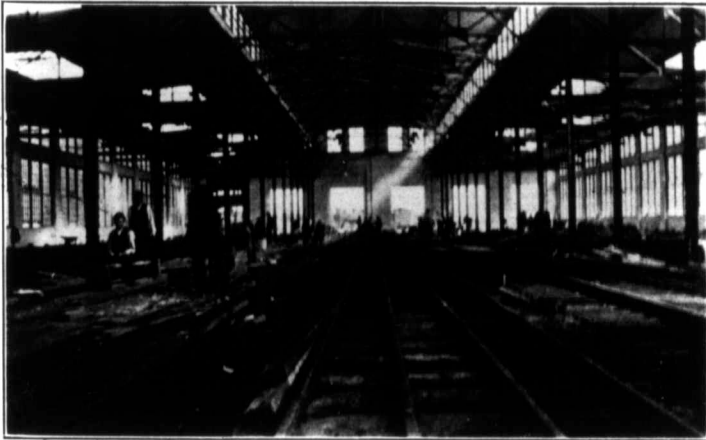
Interior of Freight Car Shop.
