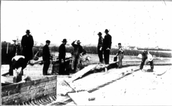
Roof, Freight Car Shop.
