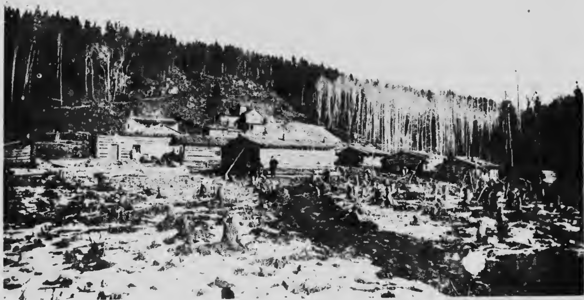
WEST END MINE
