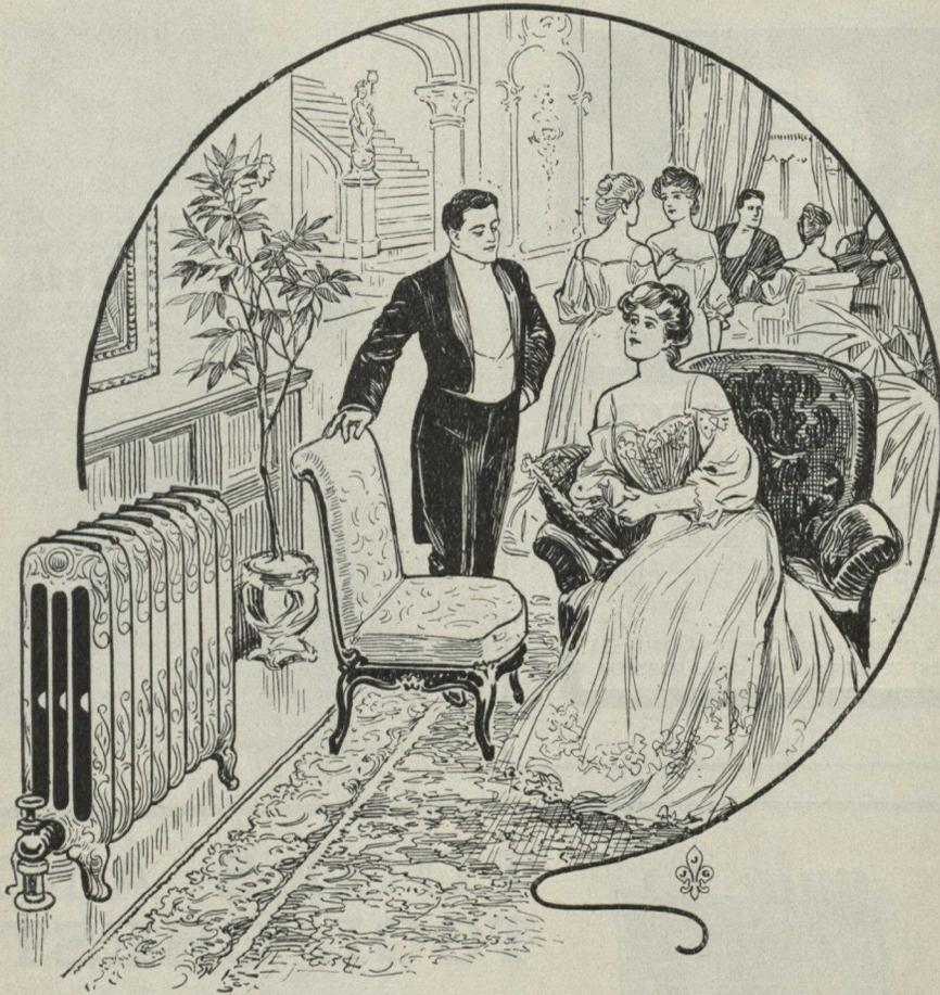
The Oxford Hot Water System of heating operates with perfect silence, as the Oxford Radiators are planned to give a clear passage for the water. They do not contain diaphragms or other obstructions in the water passages to check the water and cause the system to be noisy.
