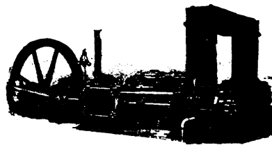
Cross-Compound Corliss Compressor
