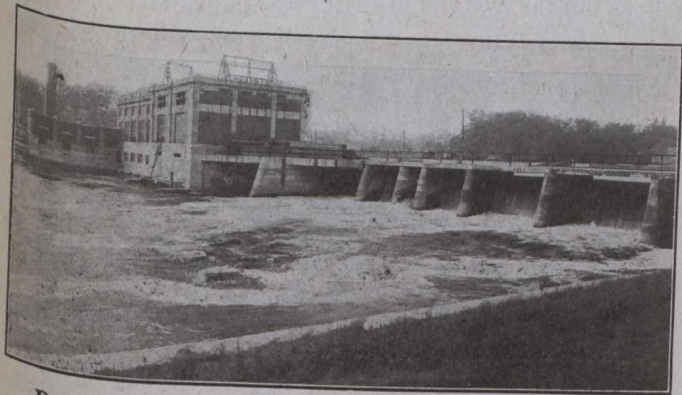
Reinforced Concrete Dam Across Otonabee River.
