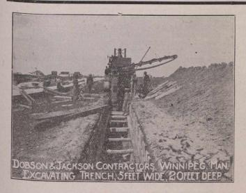
is guaranteed to work most economically and satisfactorily in any kind of soil (except rock), cutting any width from 28 to 78 inches and any depth to 20 feet, with one set of buckets, no change of parts.
