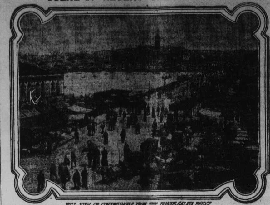
PULL VIEW OF CONTINUING FROM THE PAVILION, GALAXY BUILDING
