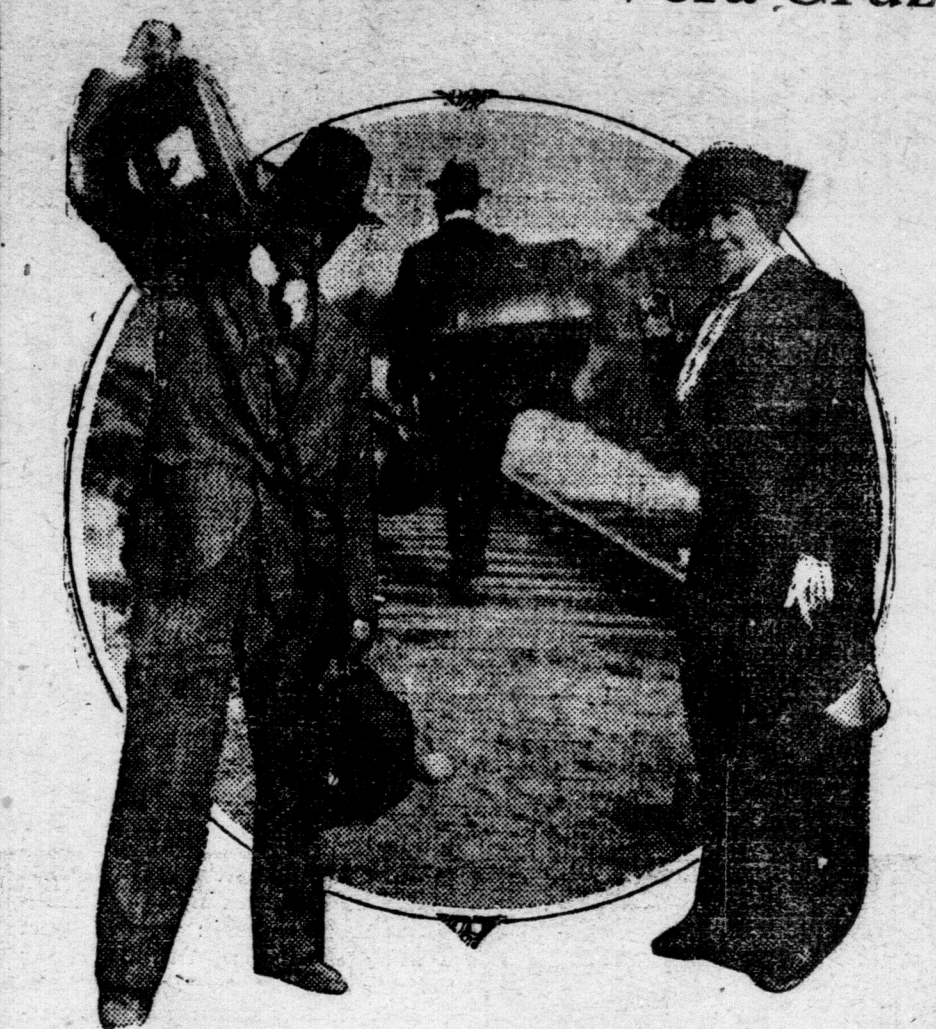
Three miles of this railroad track was torn up by the Mexican federals who fled from Vera Cruz at the time our blue jackets landed. The above picture shows American refugees walking along the railroad toward the point where the American train was waiting.
