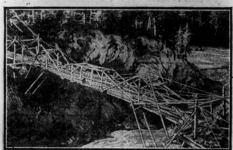
Telegraph Wire Left by Overland Pioneers Was Used by Indians to Build This Remarkable Structure.
