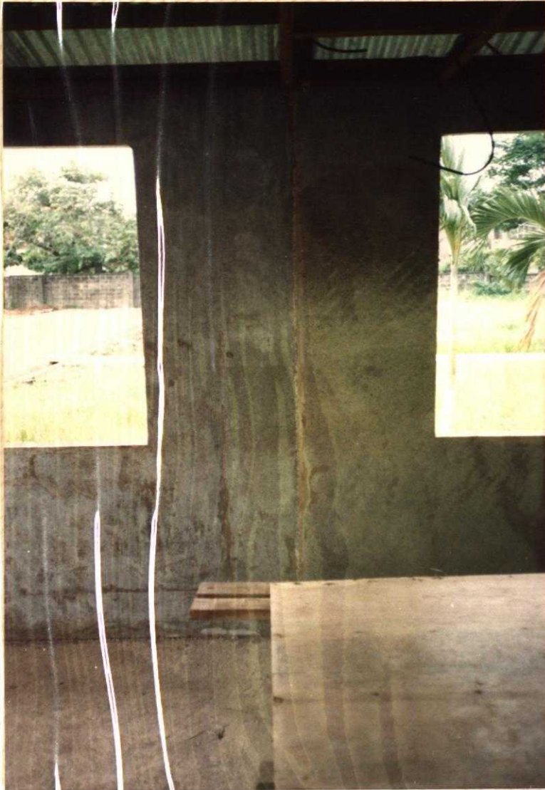
No. 44. Interior showing joint between 2 pre-cast MKL-33 wall sections.
