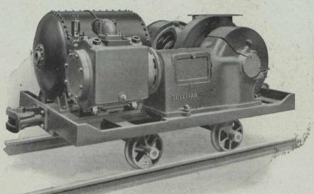
mounted on a mine car and motor - driven; maximum efficiency is gained by moving the compressor about the mine with the drill. Hundreds of these Sullivan Portable Drilling Rigs are in use to-day. Why not try one in *your* mine?
