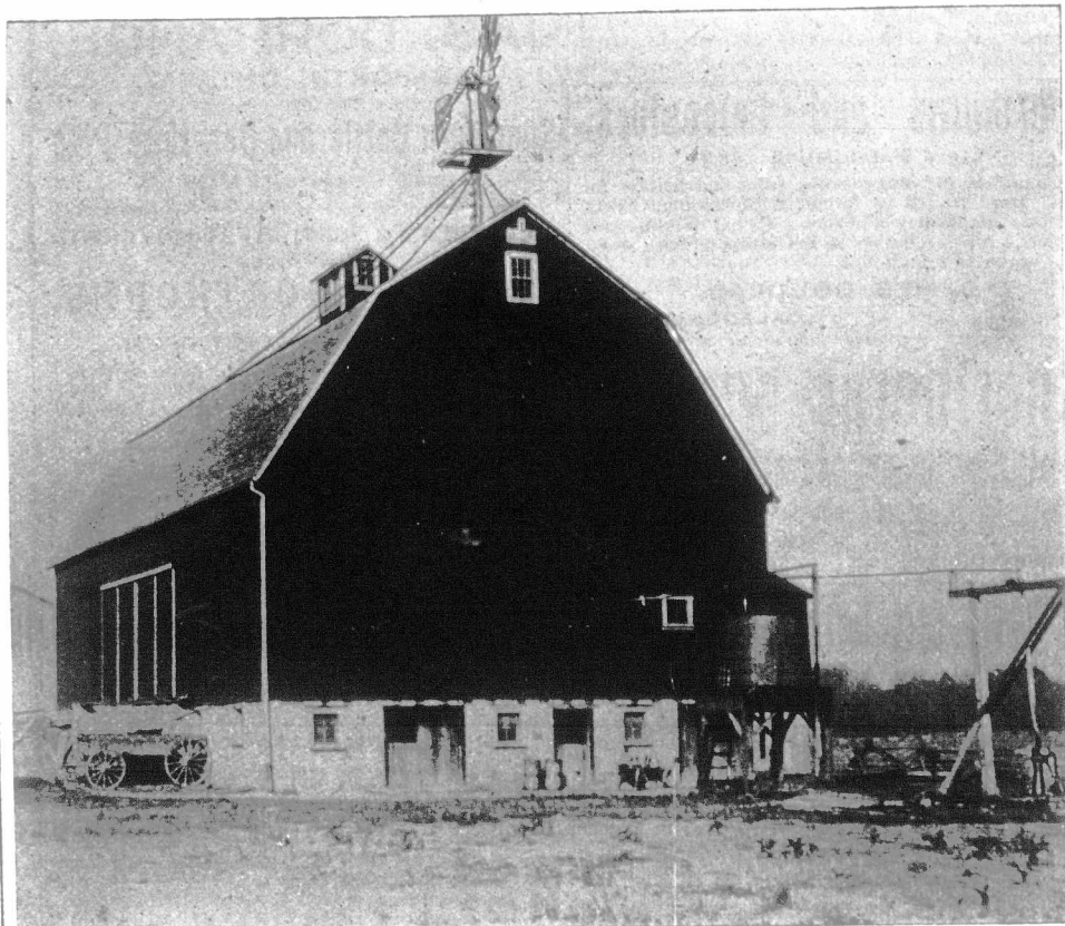
Stock barn of Mr. John D. Ferguson, in the township of Yarmouth. Dimensions of the building, 80 x 48 feet; foundations of concrete, 2½ feet deep. Floors and root cellar all of Thorold Cement.
