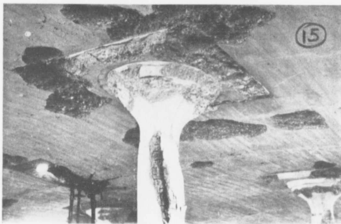
Fig. 12. A column failure.
