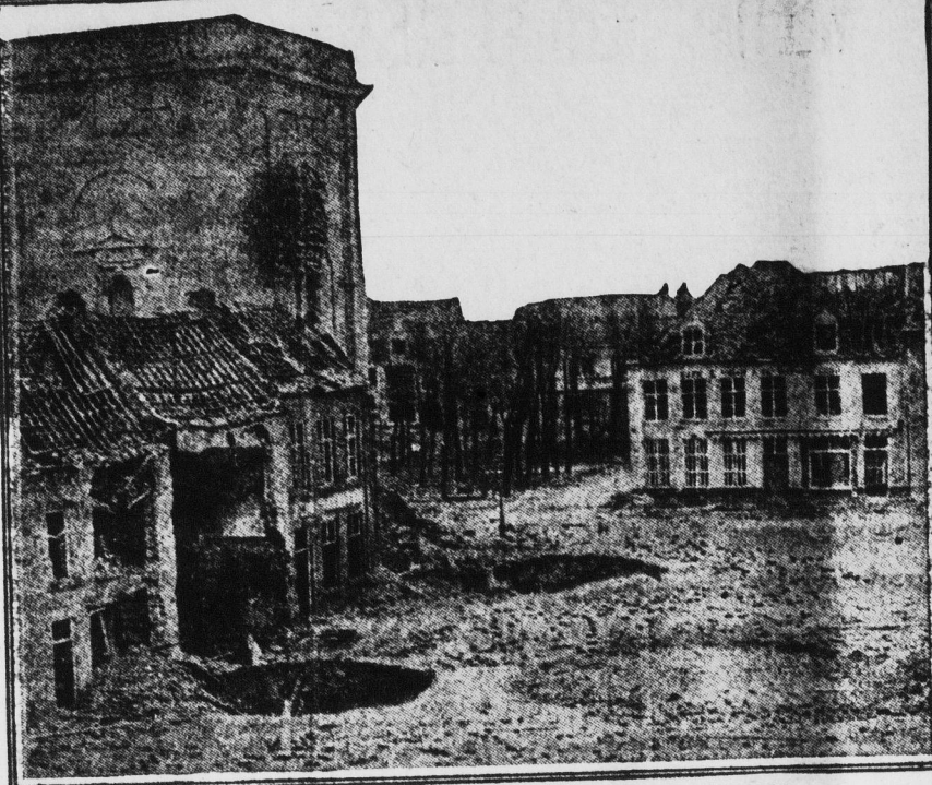
SHELL HOLES, 17 FEET ACROSS, CAUSED BY BURSTING SHELLS. The results of the continuous bombardments along the fighting line in France and Belgium may be observed at nearly every point where artillery fire has taken place. At many places the roads are seamed with "Jack Johnson" holes—grim reminders of former fighting. Time and again when burrying across the desolate no-man's-land holes—grim reminders of former fighting. Time and again when burrying across the desolate no-man's-land holes—grim reminders of former fighting. Time and again when burrying across the desolate no-man's-land holes—grim reminders of former fighting. Time and again when burrying across the desolate no-man's-land holes—grim reminders of former fighting.
