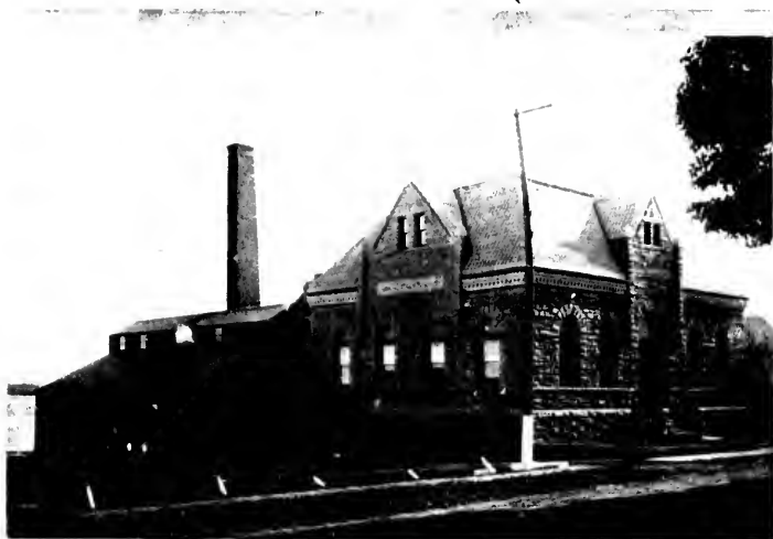
Waterworks Pumping Station.
