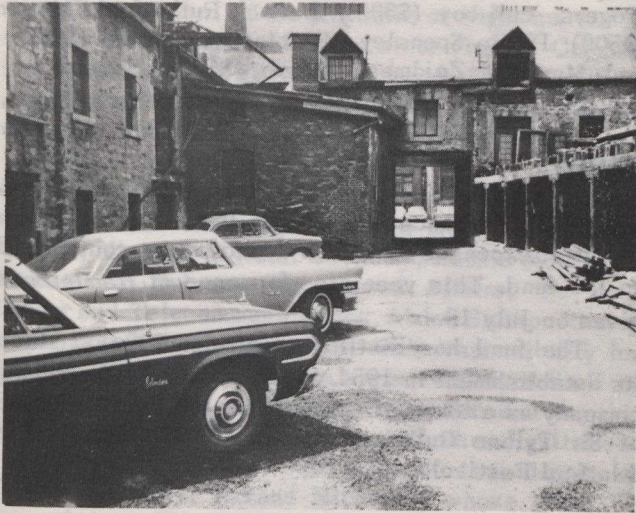
Condition of Stables before the restoration work started.
