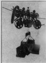
CABLEWAY EXCAVATOR AND NEAR VIEW OF GRAB BUCKET ON WELLAND RIVER SECTION
