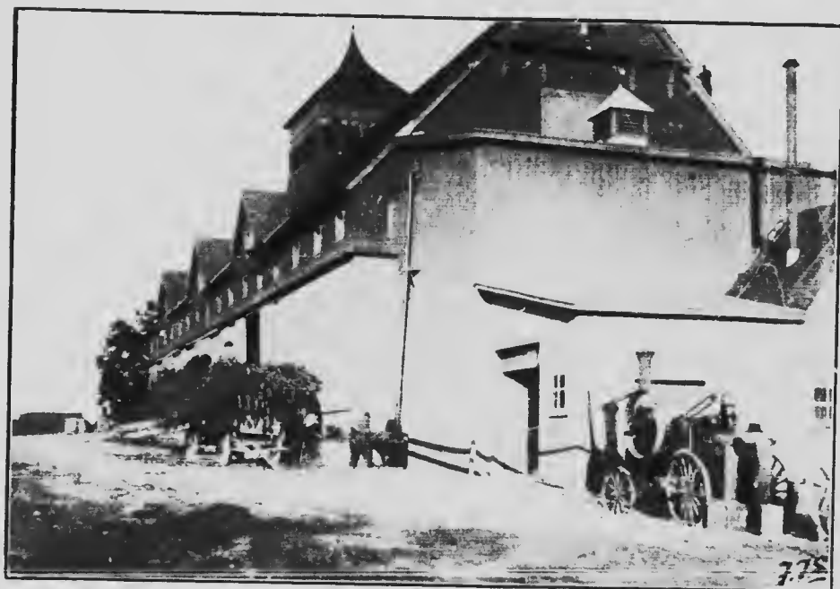
No. 10 Cutting into the Silo.
