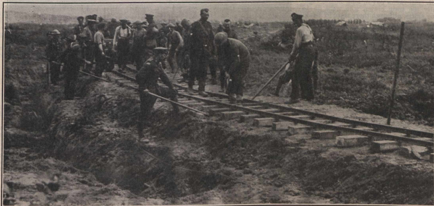
Track Gang on Light Railway Construction.
