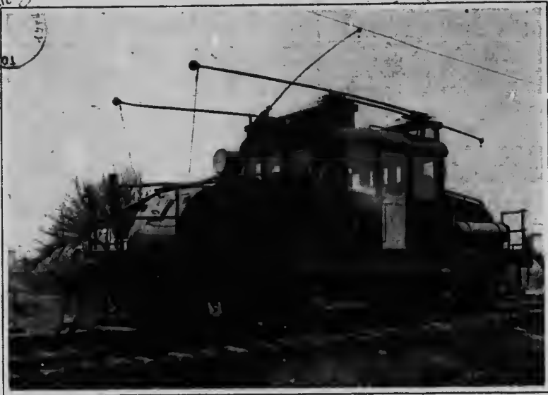
One of the electric locomotives. Note the double trolley arrangement, two poles on each side
