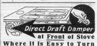
No reaching across a hot stove and over steaming pots to turn direct-draft damper on Sask-Alta. It is placed right at front of stove (see illustration) where a child can readily operate it.
