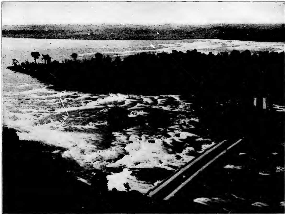
BRIDGE TO GOAT ISLAND. —The Bridge to Goat Island is one of the sights of Niagara. It is a beautiful structure, and takes the place of several previous crude wooden affairs that served as passageways in the past three-quarters of a century. The first bridge was erected in 1817. It was carried away by the ice the following spring. Other bridges were erected in 1818, 1839, 1849 and 1856. The piers were formed first by building a massive abutment of timber on the water's edge, from which were projected enormously long and heavy beams of timber. These were secured by great piles of stone, and their outer ends rendered steady by stilts thrust into the bottom of the river. A platform was then built, loaded with stone and sunk, and on this a pier was built.
