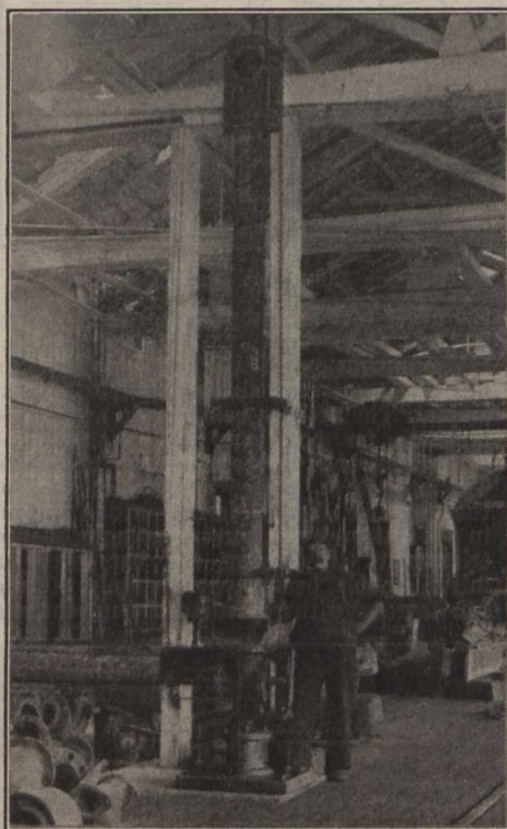
Fig. 1.—Dry Pipe Mounted for Grinding in.
