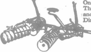
One Harrow is Out Throw; the other is In Throw. They are simply constructed, rigid and durable. The Gangs are flexible and the Disk Plates are so designed that they "hang" right into the soil. Bissell Harrows are built in sizes and weights suitable for horse or tractor use. Write Dept. W for free catalogue.
