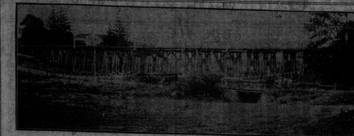
Trestlework built by Niagara, St. Catharines and Toronto Railway over Ten Mile Creek at Port Weller. This structure will be replaced by a swing bridge when the canal is completed.
