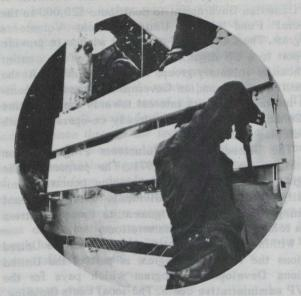
The first sign-blades go on about 1.30 p.m. They must be handled carefully so as not to scratch or damage the daymark coating. Blades are assembled in twos and threes on the ground, raised into position, bolted onto sign-blades above and slid carefully into side-rails.
