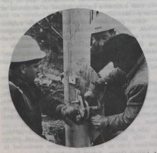
The next simple, but very important stage, is to attach the winch used to hoist up the daymark sign-blades, also of aluminum, which will eventually be used to raise and lower the complete daymark panel assembly for maintenance.
