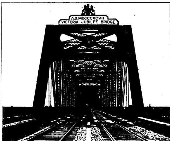
PORTAL VICTORIA JUBILEE BRIDGE.
