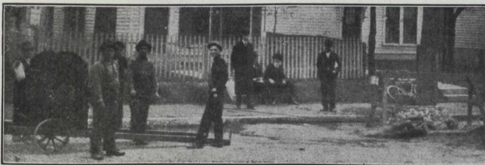
Fig. 2.—Method of Drawing Cleaner Through Small Water Mains.
