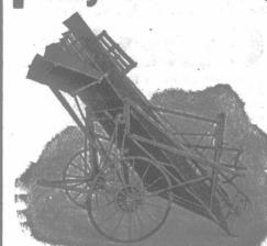
Easiest attached. Easiest det\*ched. Easiest to load from. Widest loader built. Bakes absolutely clean from swath or winrow. Doe n't pull any hay back off the wagon. Pushes the hay forward on the load Has an adjustable gate for windy weather.
