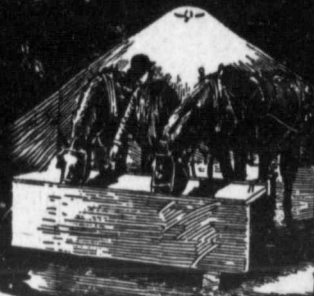
Pumps the Water
