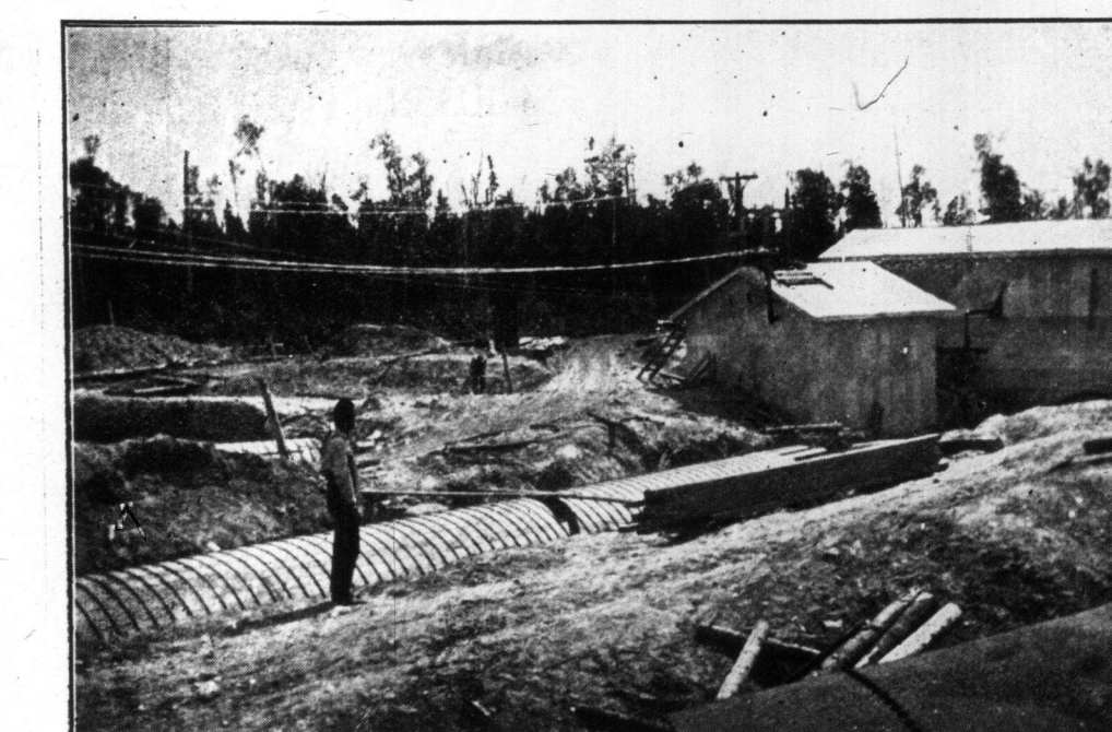
Housing Over Valve on Wooden Stave Pipe, and Over Intake at Canal Entrance, Wawaiten.
