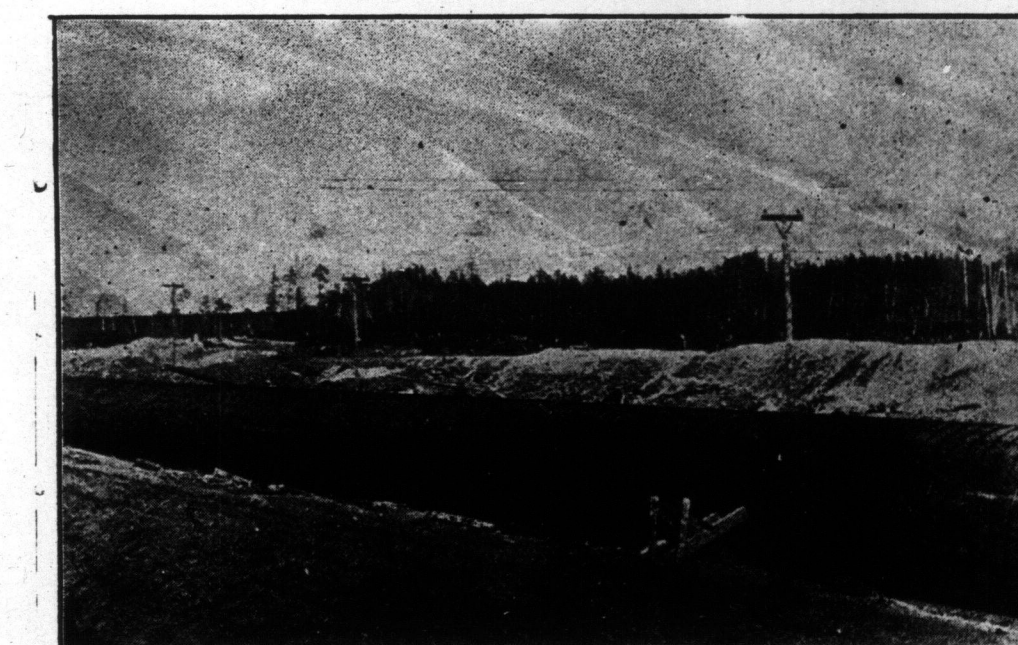
Portion of Wooden Stave Pipe at Wawaiten Before Back Filling With Sand and Clay.
