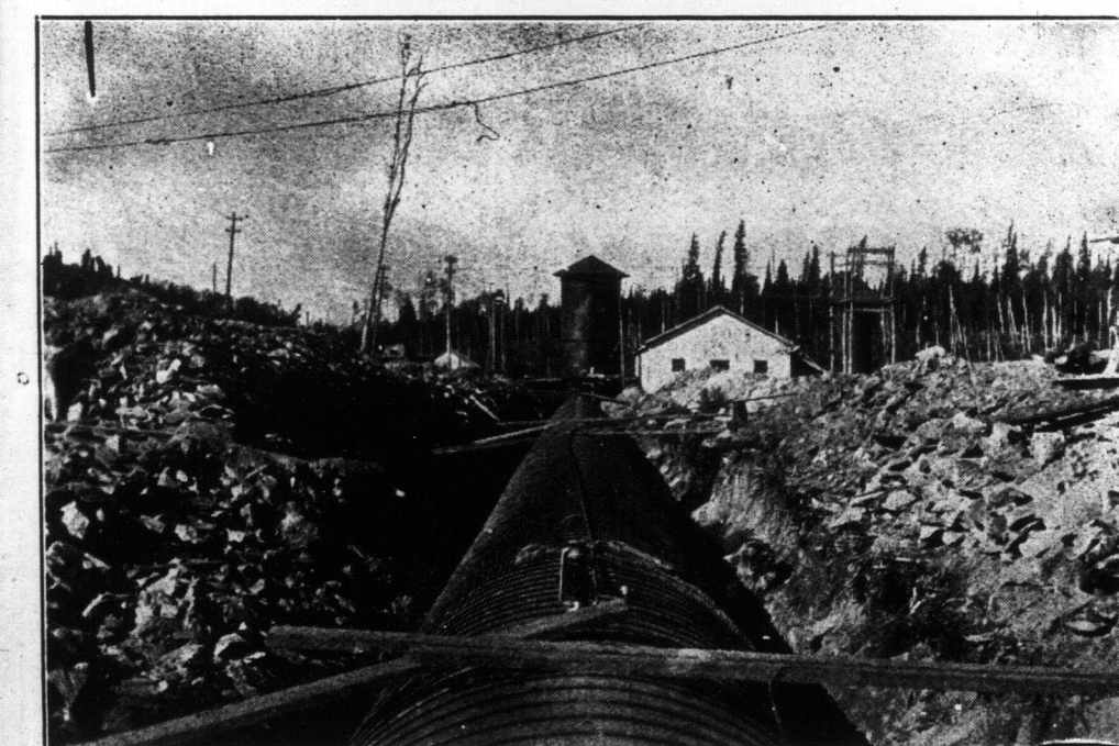
Installation of Nine-Foot Wooden Stave Pipe at Sandy Falls.
