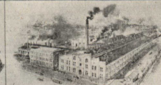
NEW FACTORY BUILT IN 1895 SINCE THEN THE FOLLOWING EXTENSIONS HAVE BEEN MADE. MACHINE SHOP LENGTHENED 140' NOW 440' x 170' BOILER SHOP 100' NOW 220' x 80' (WITH CORRESPONDING MOULDING SHOP 100' NOW 180' x 80' (WITH CORRESPONDING BLACK SMITH SHOP 80' NOW 100' x 40' IN EQUIPMENT.
