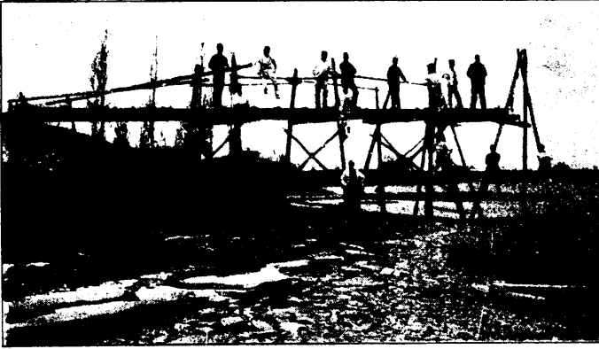
A BRIDGE IN COURSE OF CONSTRUCTION.
