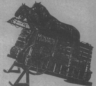
The McGILL MONARCH TREAD POWERS are the best general-purpose Farm Powers on earth, and are the only Powers made having Angle Steel Track, Cold Rolled Steel Shaft, 7-inch Travellers, Solid Maple Lags, with Brake entirely independent of Band Wheel. A patent Governor or Speed Regulator with each Machine. Write for prices.
