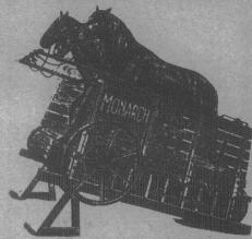
The McGILL MONARCH TREAD POWERS are the best general-purpose Farm Powers on earth, and are the only Powers made having Angle Steel Track, Coid Rolled Steel Shaft, 7-inch Travellers, Solid Maple Lags, with Brake entirely independent of Band Wheel. A patent Governor or Speed Regulator with each Machine. Write for prices.
