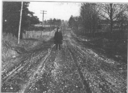
A New Road in Marked Contrast to the one finished with a Roller
